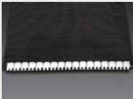
1) Square the belt end and place the fastener adapting it to the thickness of the belt
