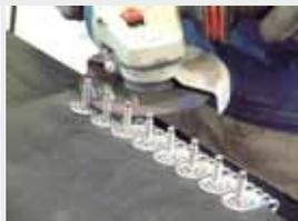
3) Use an angle grinder to remove excess bolts
